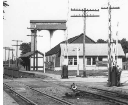
John Young's coal yard, which incorporated the pickle shop's management house and part of the old factory.
